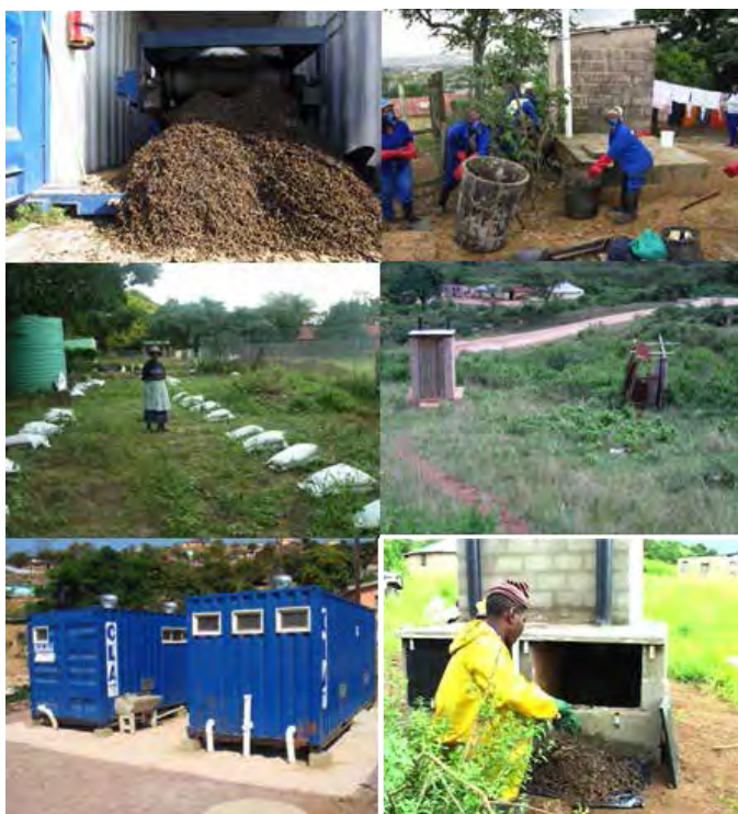
Sanitation systems in eThekweni (clockwise from top left): LaDePa pelletizer; VIP emptying; UDDT and traditional pit latrine; emptying of UDDT vault; community ablution blocks; reuse for agriculture.
