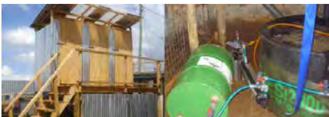
One of the three complete system and superstructure deployed in Eldoret, Kenya (left) and contained treatment system below (right). Each system comprises of three toilets, one anaerobic digester, and one heat sterilization system. All systems are self-contained.
