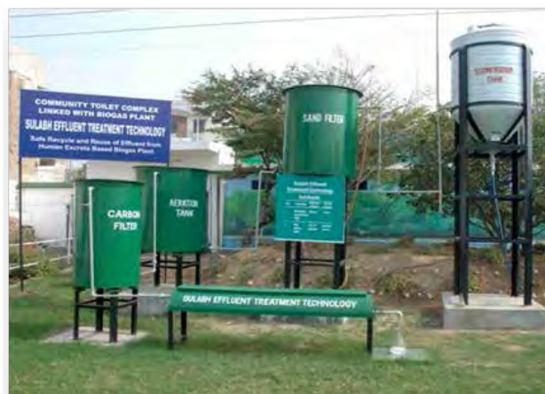
Sulabh Effluent Treatment System (SET)
